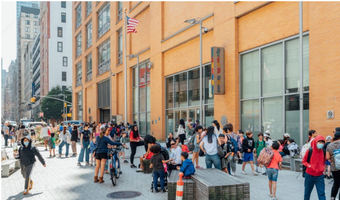
Figure 2.3A Spruce Street School, New York, USA - Generous sidewalk drop-off area, clear signage and visibility into the school lobby
