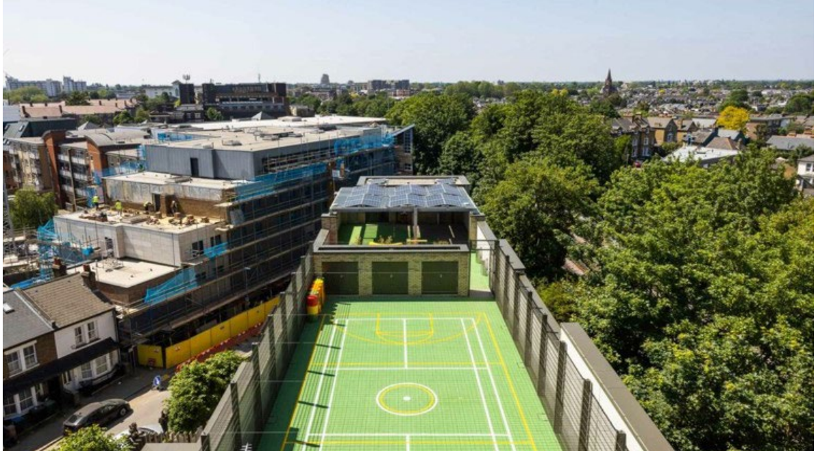
Figure 3.5.2A Kingston Community School, UK - A Rooftop playground with high guards
